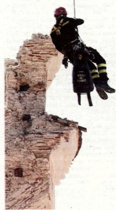
A church being inspected. Four have been damaged very badly
